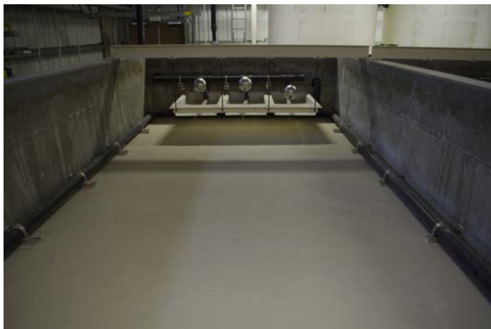
Figure 15. Filter cell before commissioning.
