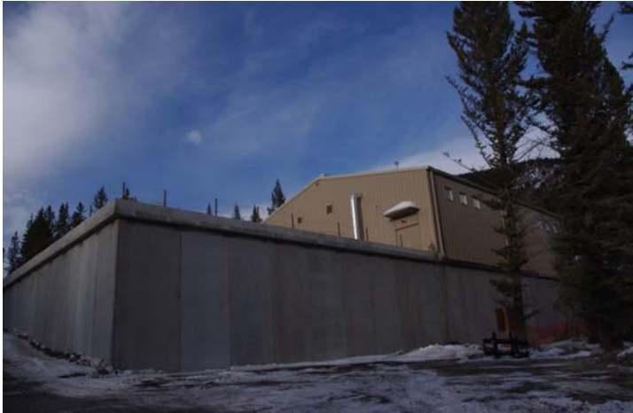
Figure 12. Water treatment plant located on top of treated water storage.
