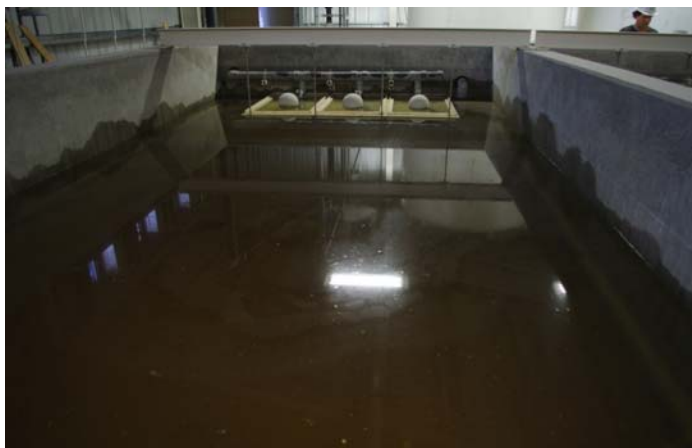
Figure 15. Filter cell before commissioning.
