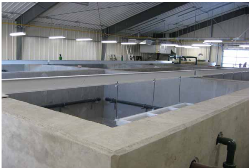
Figure 10. Interior view of water treatment plant showing filter cells.
